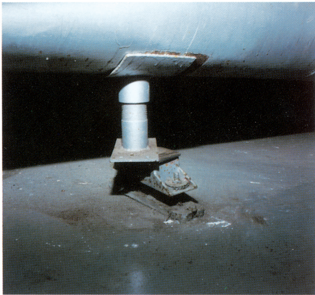
Figure 6. The attachment of the stand to the pipe and to the top of the machinery mount is not proper. This allowed the stand to shift off the mounting (basement location, 6 stories, approximate seismic excitation - 0.3 g horizontal, 0.25 g vertical).
