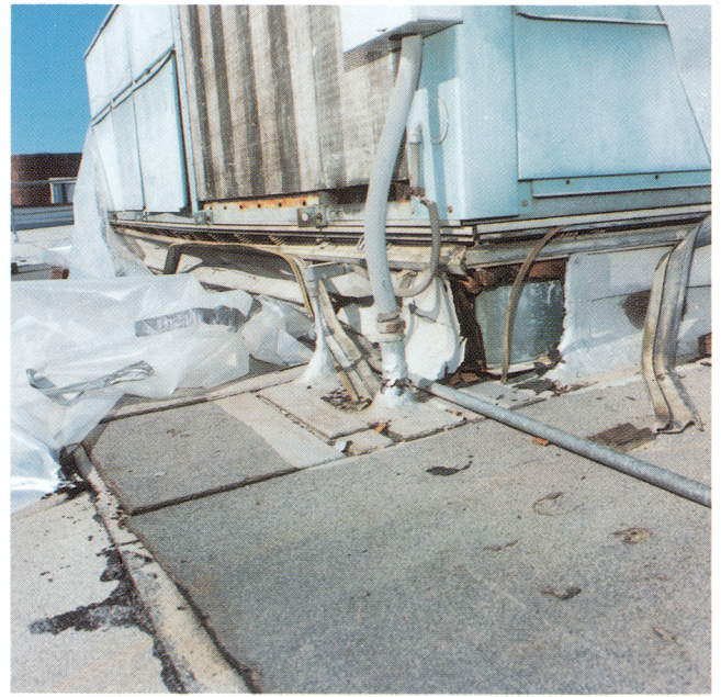
Figure 16. Isolated aluminum roof curbs failed because of the lack of structural strength of the aluminum sections (roof location, 4 stories, approximate maximum seismic excitation - 0.3 g horizontal, 0.22 g vertical).
