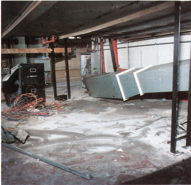
Figure 12. Duct failure resulted when sway braces were omitted (4th floor location, 4 stories, approximate maximum seismic excitation - 0.4 g horizontal, 0.28 g vertical).
