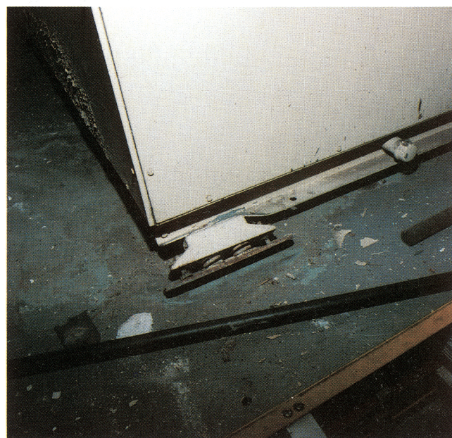
Figure 5. Direct mounting of vibration isolators can result in failure if the machinery frame is not adequate and local buckling occurs (roof location, 2 stories, approximate maximum seismic excitation - 0.42 g horizontal, 0.3 g vertical).
